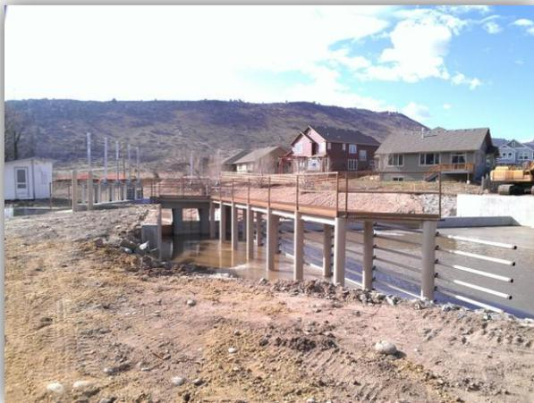
**Figure 3 – Repaired ditch company diversion and headworks**
