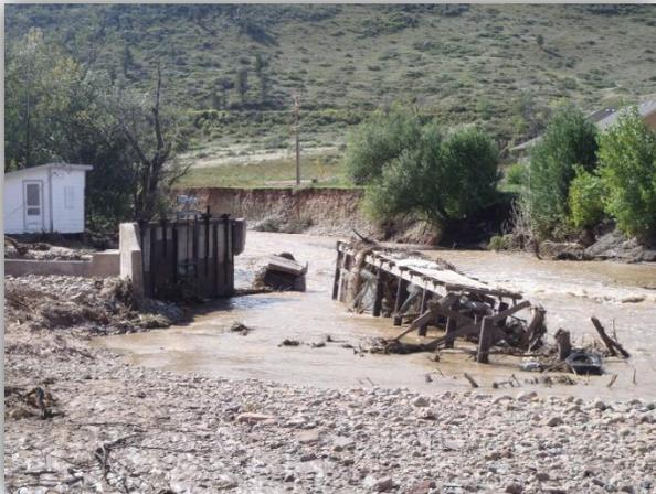
Figure 2 - Destroyed ditch company diversion and headworks
