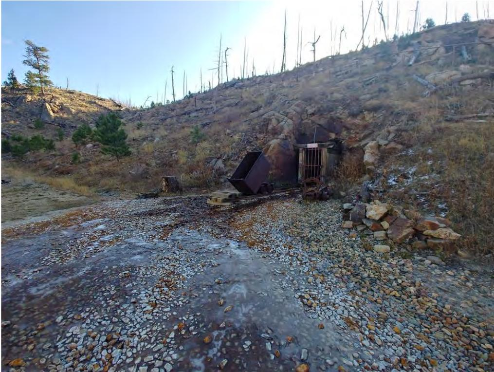
Figure 2. Draining adit at the Duval Mine. Adit waters flow across, and infiltrate into, mine wastes before reaching Castle Gulch below.
